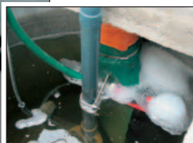
Implementation of a submerged pump for the water supply of Coolbox
