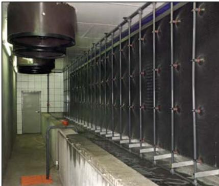
Nozzle groups spray water on to the front of the filter bank so that dust cannot cling to the filter.
