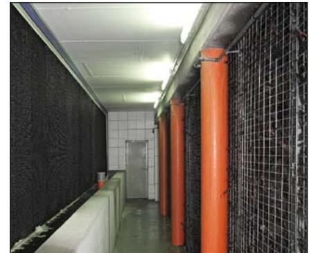
The third cleaning stage consists of root timber and is used for the microbial transformation of odour-carrying agents.
