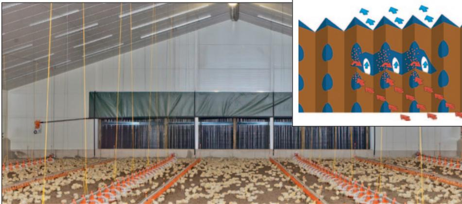
Use of the StuffNix dust filter in a broiler house – qualified measurements determined a total dust separation rate of up to 70 % and a separation rate of fine dust of 32 %.
