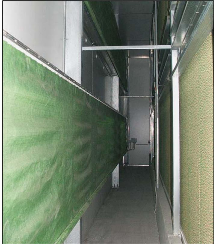
Tunnel inlet with roller curtain
