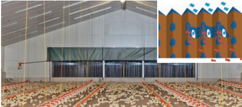
Use of the StuffNix dust filter in a broiler house – qualified measurements determined a total dust separation rate of up to 70 percent and a separation rate of fine dust of 32 percent.
